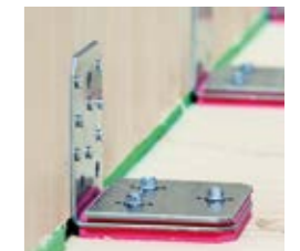
Inset joint, full-thread screws perpendicular from outside
