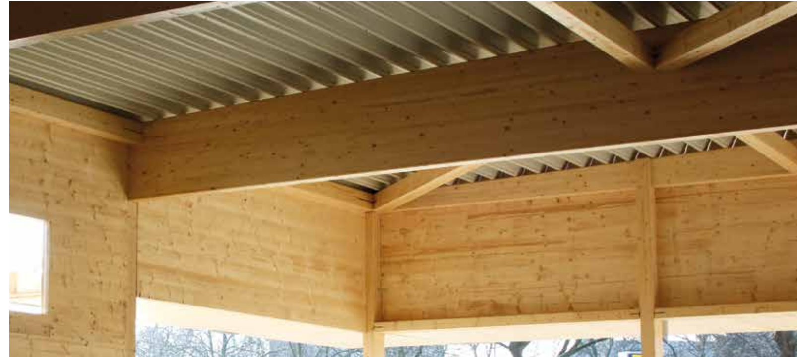
Rapid roofing will provide the best protection of visible surfaces from weathering effects.
