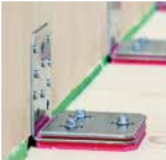
Inset joint, full-thread screws perpendicular from outside
